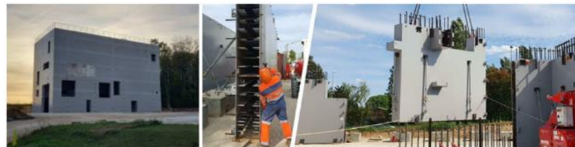
FIG. 4. Steel-Concrete modules (SCHEDULE mock-up at the site of EDF R&D in Les Renardières)
